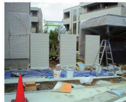
Spraying of paints 吹付け塗装
