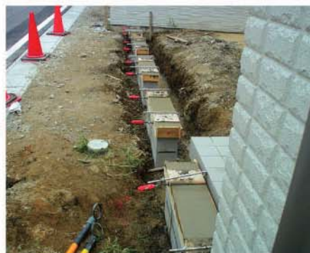
Base of structure 基礎
